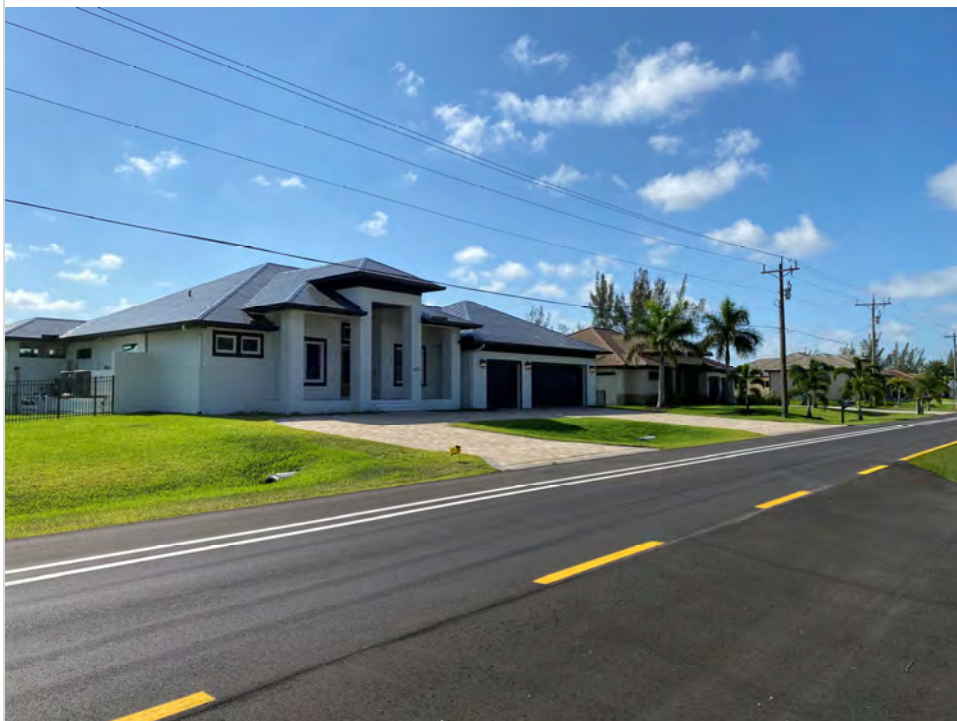
VIEW OF NEW SINGLE FAMILY RESIDENTIAL CONSTRUCTION LOCATED ALONG THE EAST SIDE OF OLD BURNT STORE ROAD
